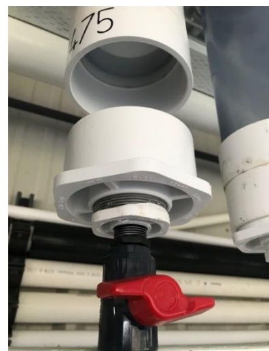
Fig 20. Detail of reducer coupling and valve. Reducer slip fits into the base of the coupler with screen.
