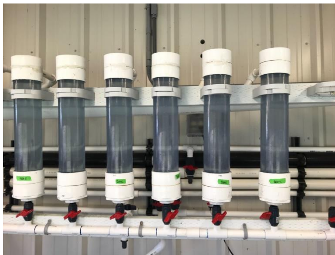
Fig 22. Multiple combined setting/primary nursery cylinders attached to wall in the Pacific Hybreed laboratory facility.
