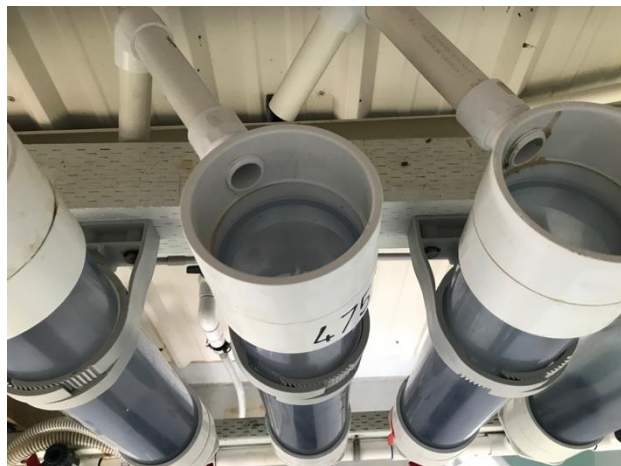
Fig 21. A view of the top of the combined setting/primary nursery cylinder system. Note the exit pipe to a common gutter used to collect outgoing flow. In this view, the couplers are fit with interchangeable 475 micron screen, used for holding one week post set seed. All connections are slip fit and require neither glues nor O-rings to maintain a watertight connection.
